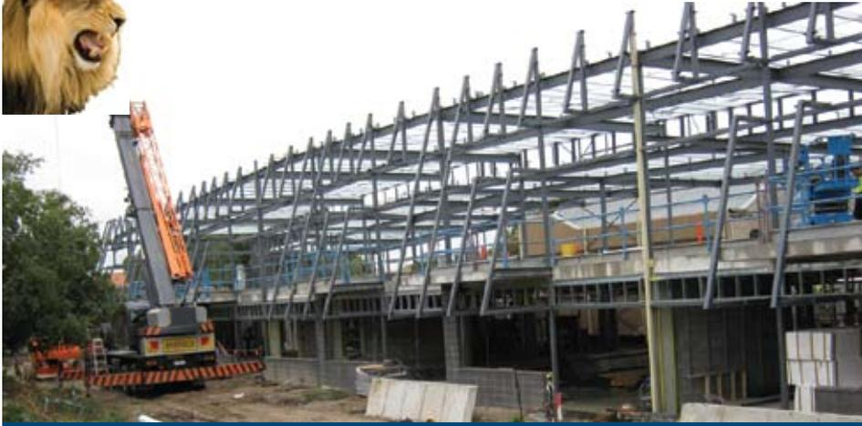
GROUND FLOOR EXTERNAL WALLS AND FIRST FLOOR SUPPORTING STEEL WORK, GANDEL BESEN HOUSE
